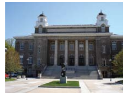
Syracuse Carnegie Library, New York, USA
